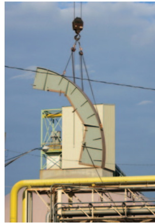
End Ring Repair Section
