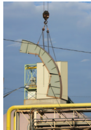
End Ring Repair Section
